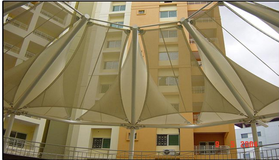
Tensile Membrane Structure Swimming Pool Cover (Interior View) Mantri Elegance Bangalore
