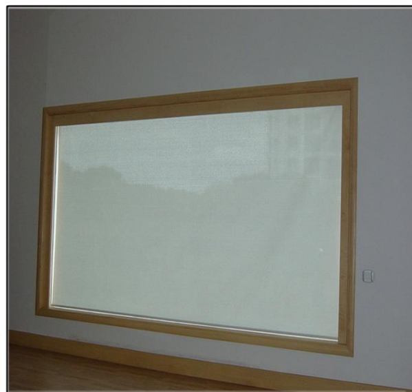
Automated Roller Blinds (Closed View) GMR MD's Residence Bangalore
