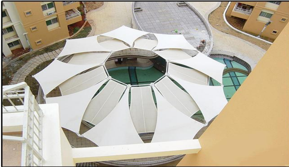
Tensile Membrane Structure Swimming Pool Cover (Exterior View) Mantri Elegance Bangalore
